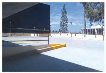
ABOVE A Since the urethane base coat from the existing coating system was usable, the Nash crew was able to save their client the time and expense of having the affected areas stripped down to bare concrete.
