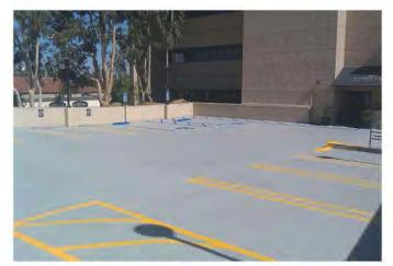
ABOVE — To compensate for faster cure times brought on by higher ambient temperatures, the crew mixed smaller batch sizes. But the coatings' quicker sets also helped the crew make up for lost time. The Nash crew installed the topcoat on a Friday, brought the striping crew in on Monday, and had the parking structure open to traffic on Tuesday.
