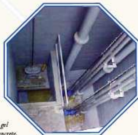
Manhole Rehabilitation USA
