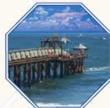
Concrete Piers Santiago, Chile
