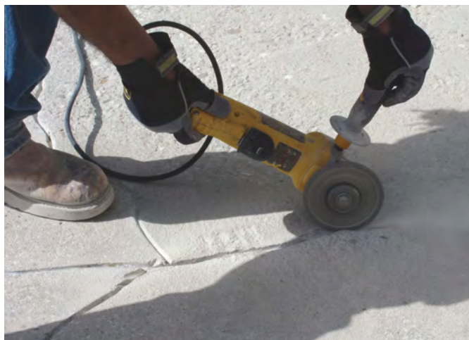
LEFT ◀ After the Blason crew finished shot blasting the deck, any cracks in the concrete were routed, primed and caulked.
