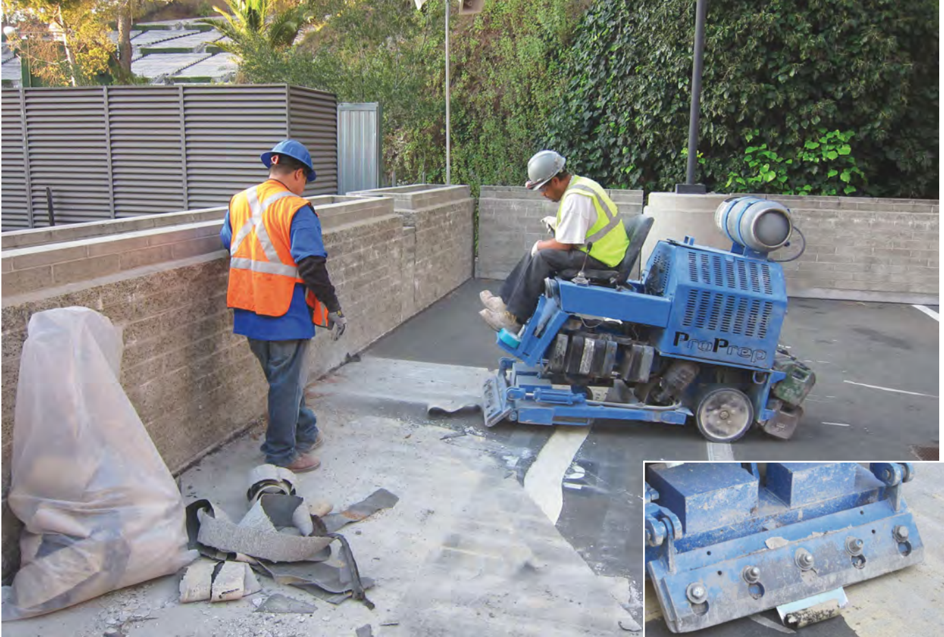
ABOVE ▲ In order to remove the failed coating, California Restoration & Waterproofing subcontracted with Blason Industries. The Blason crew used a Blastrac shot blaster among other equipment (inset) to remove the existing coating from the deck.
