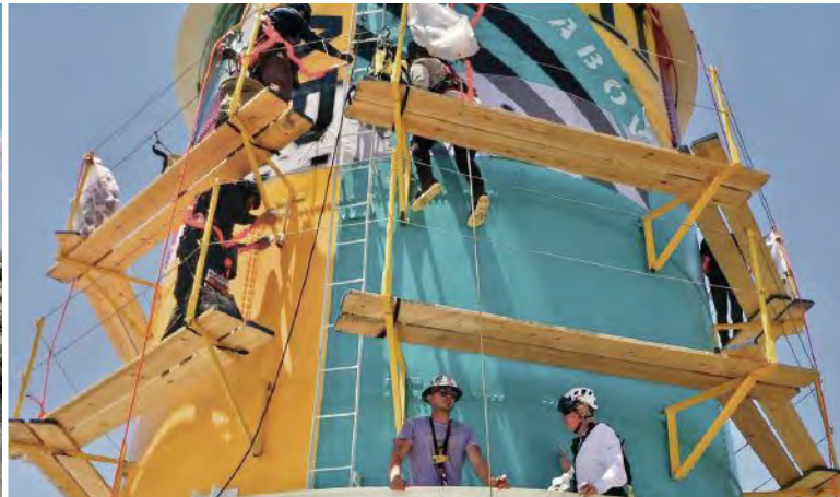
Restoring a historic water tower in Dallas, Texas, was a team effort. Lead by TankSpek, a 2–5 person crew worked on prepping and coating, while an artist gave it a decorative touch to finish.
