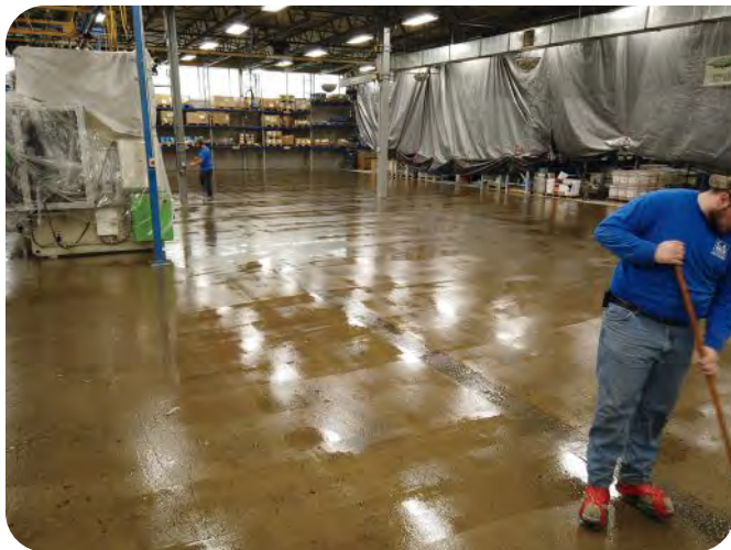
The 100 percent solids epoxy primer, #5100 clear from C.A. Reed, went down at an average of 8 mils using squeegees and 18-inch backrollers.
