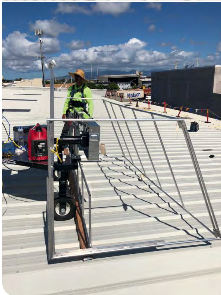
Converting a cold storage building required SPF and coatings to the rooftop and interior walls. It required covering two kinds of substrates, too: J rib and corrugated metals.
